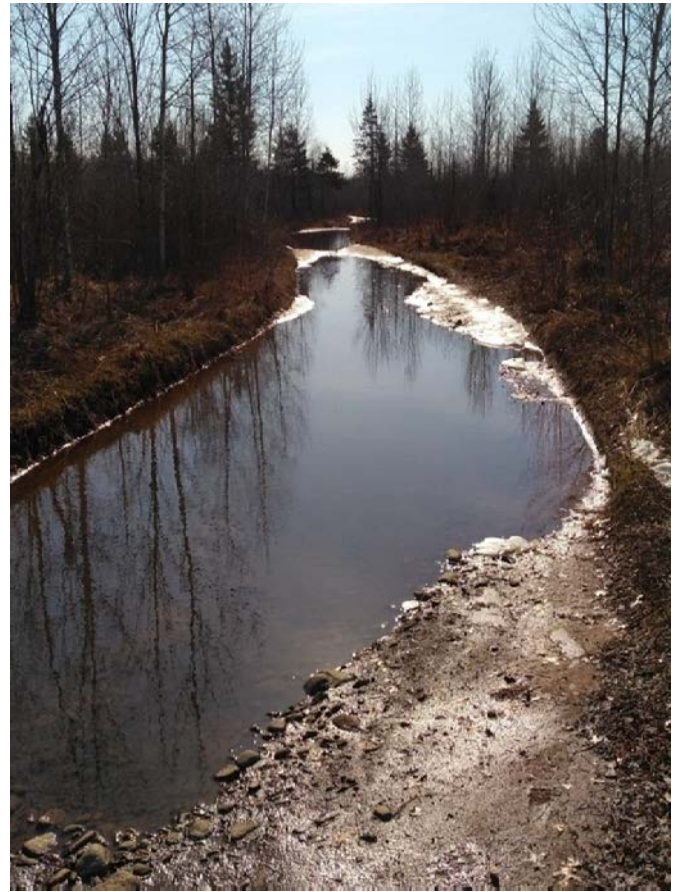
Portion of Trail in Little Rice Needing Rehabilitation
