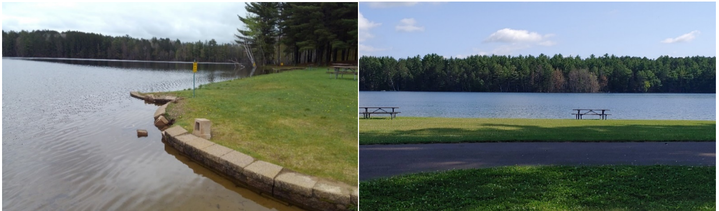
Retaining Wall and Beach Area: Almon Park, Town of Pelican
