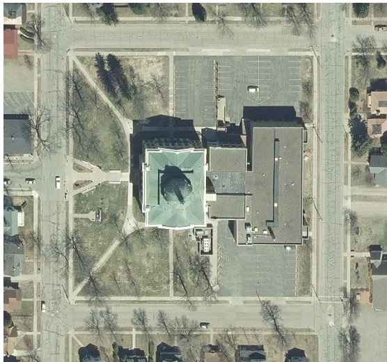
2019 Aerial Photograph – Oneida County Courthouse
