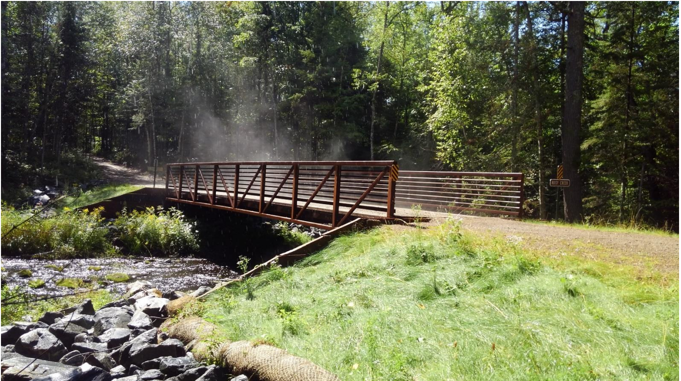
Photo of the new ATV/UTV and Snowmobile Bridge over Noisy Creek in the Town of Enterprise.
