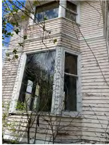
Views of typical siding damage, or siding, windows, and trim needing scraping and painting.
