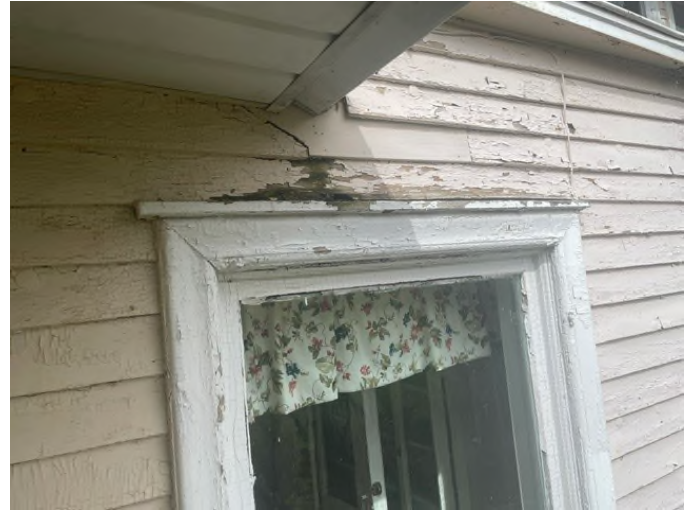
Views of typical siding damage, or siding, windows, and trim needing scraping and painting.
