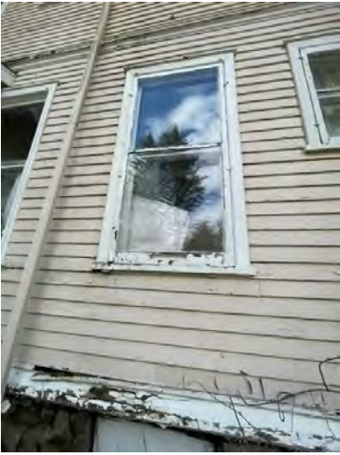
Views of typical siding damage, or siding, windows, and trim needing scraping and painting.
