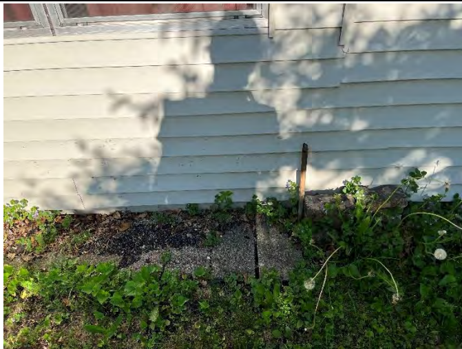
Pipe sticking up in front of house.
