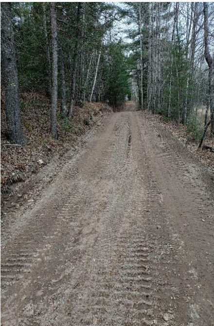
Rehabilitation Project by Rynders, Inc.
