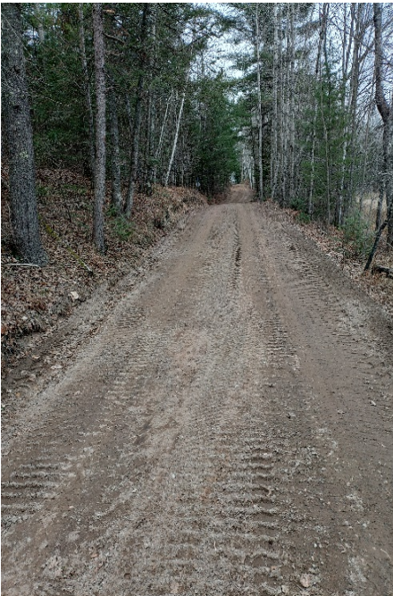
Rehabilitation Project by Rynders, Inc.
